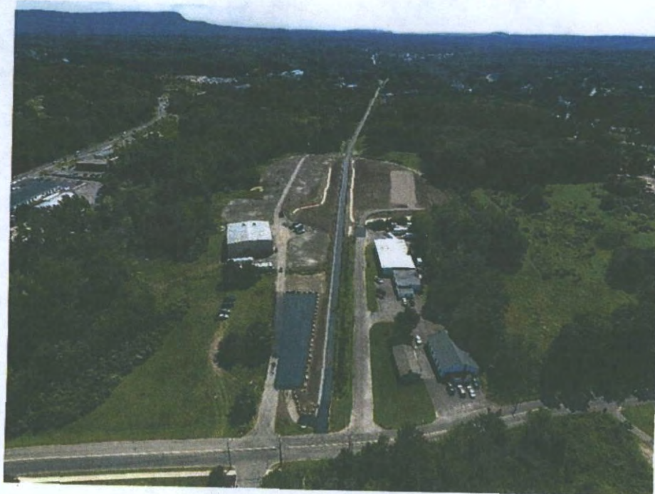
Photo 2: Cap Construction Complete (Sept 2017)
