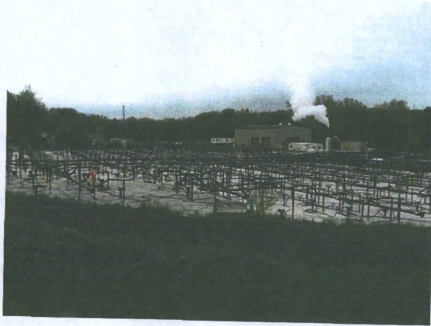
Photo 1: During In Situ Thermal Remediation (ISTR)
